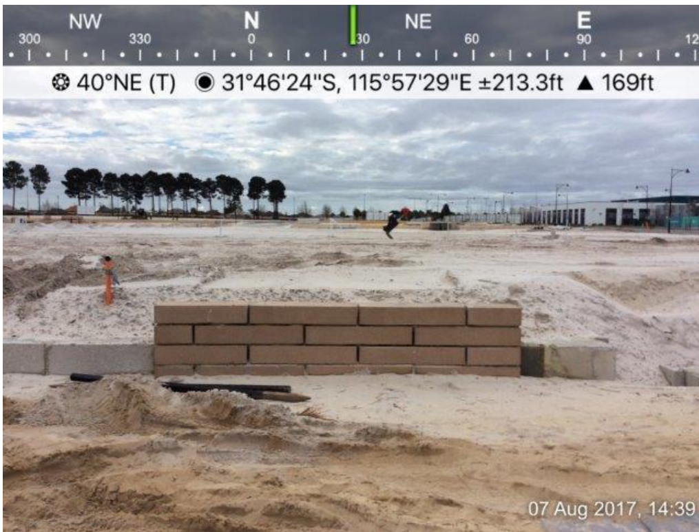
Photo 20: Off-site cleared/managed low fuel areas (excluded under Clause 2.2.3.2 e and f) east of project area
